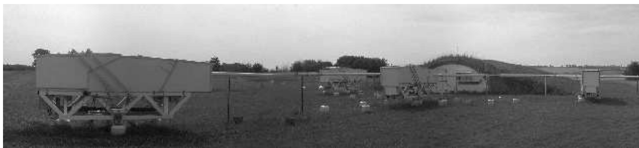
Figure 1. An exterior view of COAST in spring 2002. Four of the five telescope enclosures are visible, as is the grass-covered beam combining laboratory in the background to the right. The beampipe connected to the western-most array element extends out of the frame to the right. In this configuration the maximum baseline is \sim 45 m. The small white stumps protruding from the ground are the foundation pads for the telescopes.
